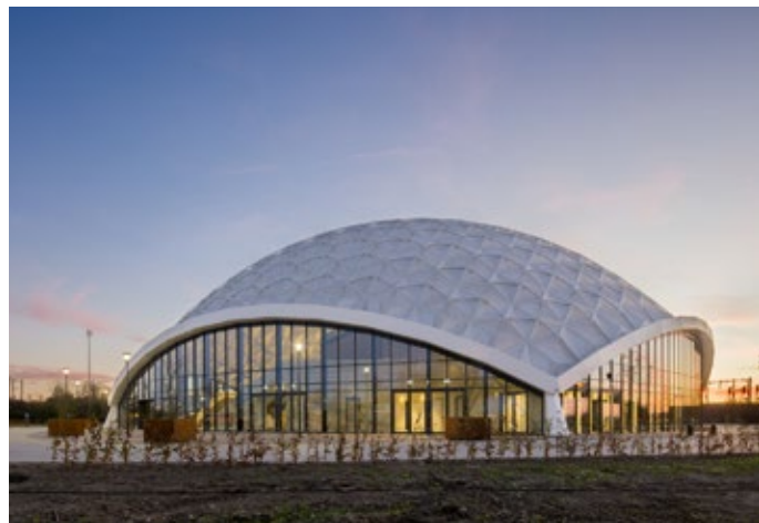
Amsterdome, Amsterdam — Architect: Architectenburo Guido Bakker — ConceptWall 50
